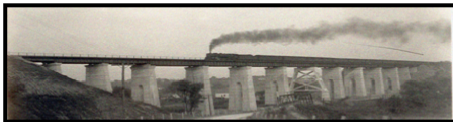
Michigan Central Railroad Kettle Creek Bridge
